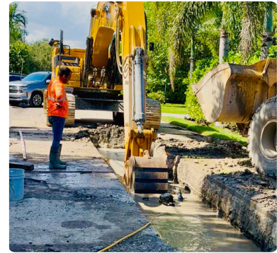
Septic-to-Sewer trenching and diving in Shores Estates NE 105 th street
